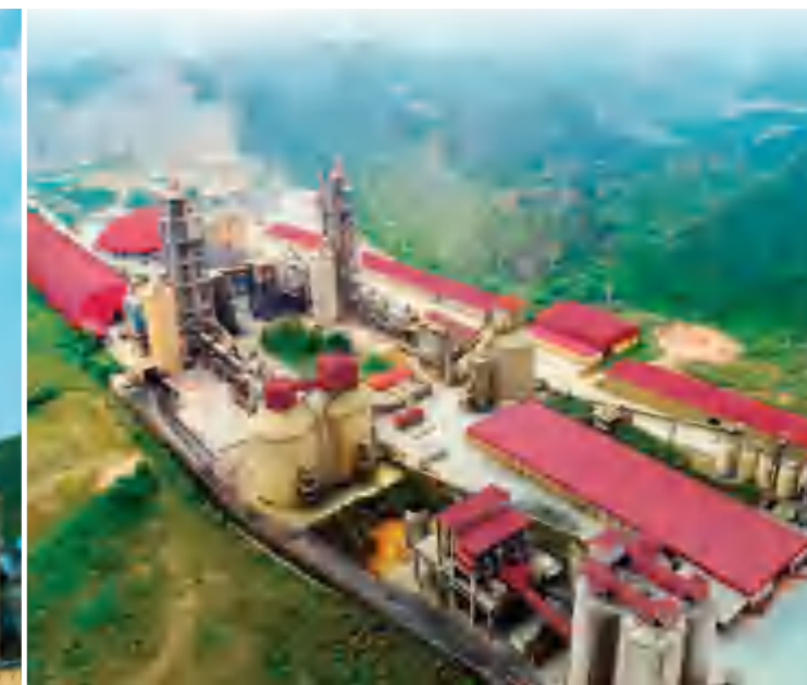
2x2,500 t/d project for Huong Duong Cement Co., Ltd. in Vietnam
