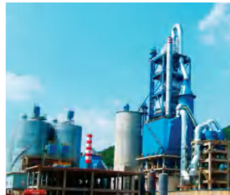
3,000 t/d new dry process cement production line project for Huirui Cement Co., Ltd. in Guizhou Province
